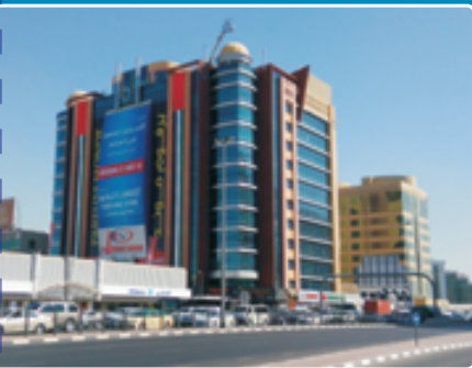
The UAE Regional Sales and Service Center
